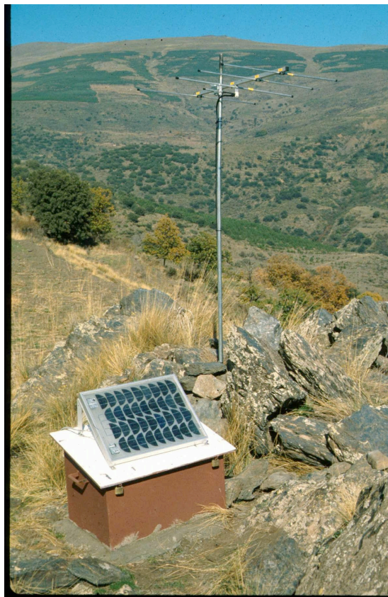
Figure 7.15 A small 12 W mono-crystalline solar panel mounted on top of the case of a temporary seismic station. Both sides of the panel is light sensitive so the roof of the case is white-painted to reflect the diffuse radiation to rear side of the panel.
