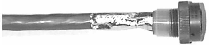
Figure 33: Wrapping foil tape around outside of the connection
