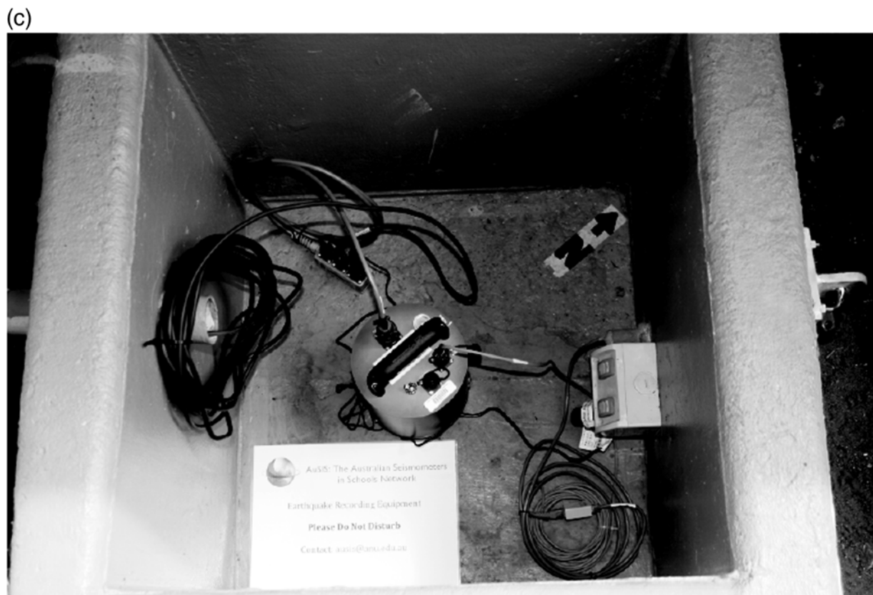
▲ Figure 3. Types of installations: (a) seismometer installed in crawlspace beneath building and on a concrete pier, (b) standard installation of seismometer directly sitting on a concrete floor, and (c) impressive seismic vault built by the construction class at a school.
