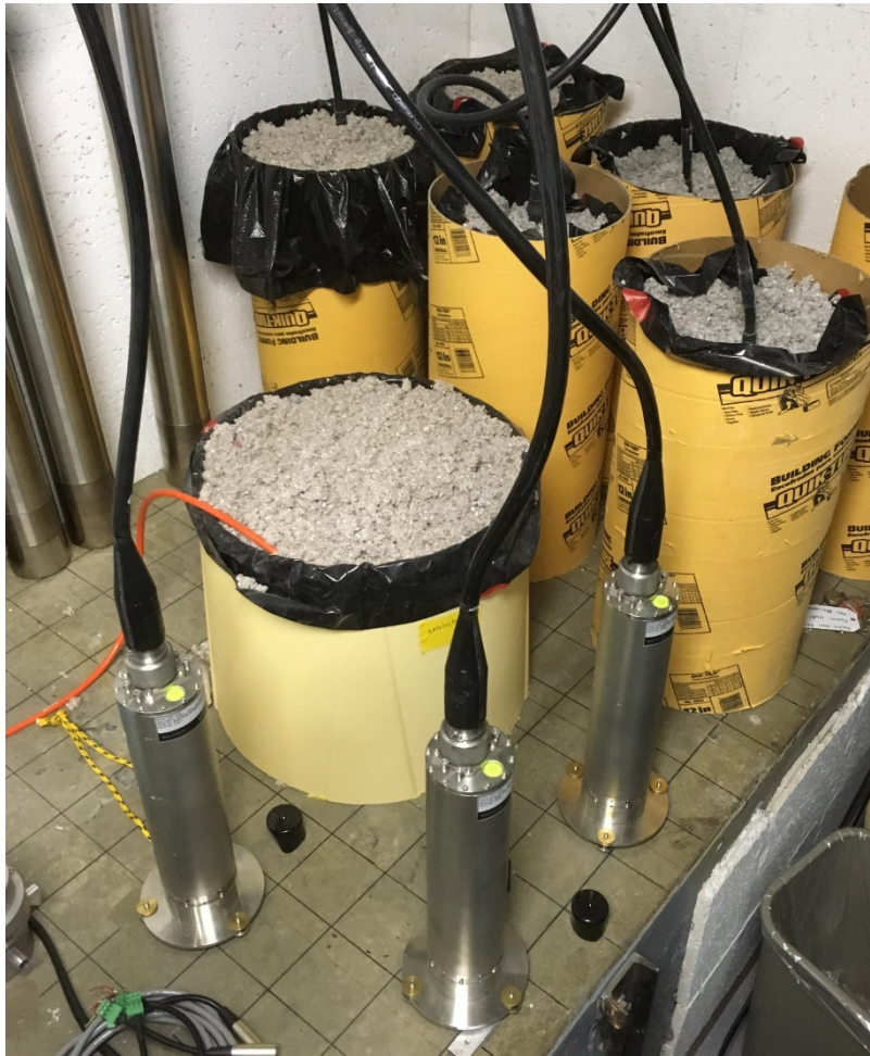
Figure 5 Picture of installed Seismometers
