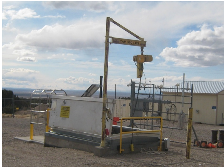
Figure 2 FACT Site Bunker
